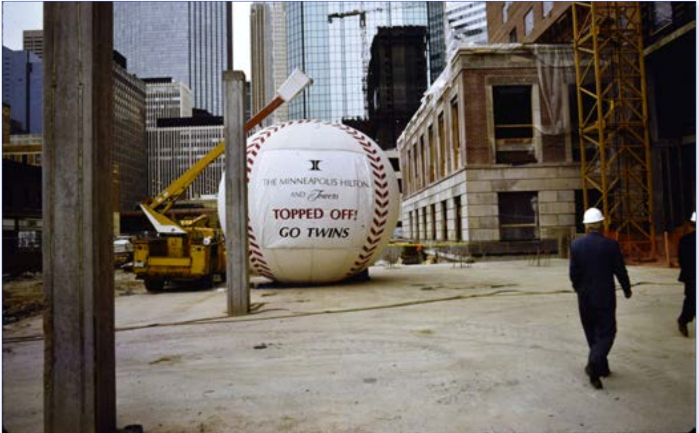
The topping off ceremony marks the completion of a building's framing during the construction process. Taken during the Minnesota Twins successful pennant year, 1991. Credit: Hennepin County Library
